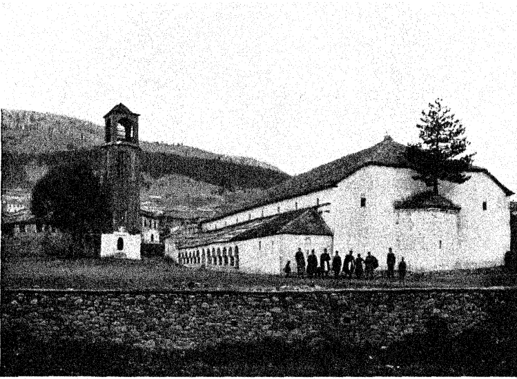
1. EXTERIOR FROM THE EAST
