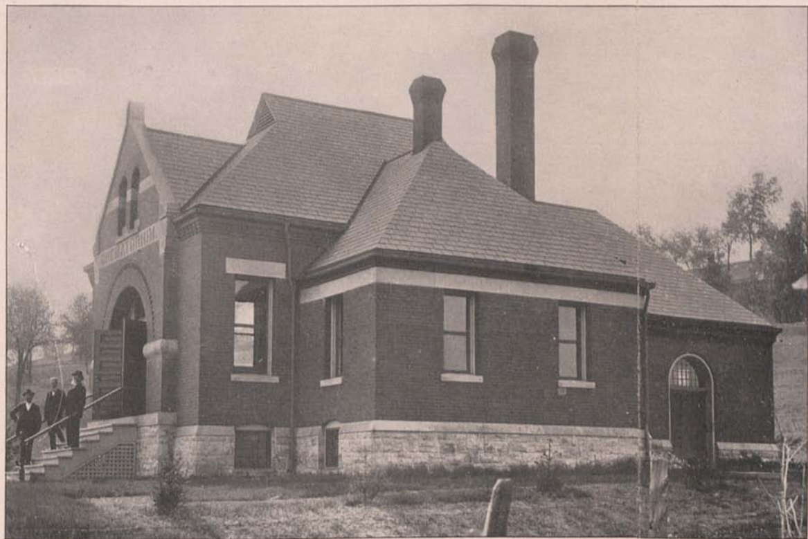
DAVENPORT CREMATORIUM — SOUTH-EAST VIEW.
