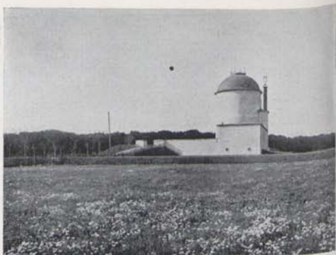
The Peace Temple in Helsingborg, seen from north-east. The first stage.
