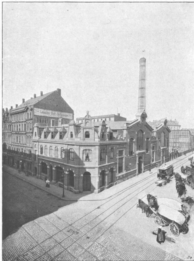
LEIPZIG, Kraftstation — Station centrale — Power station.
