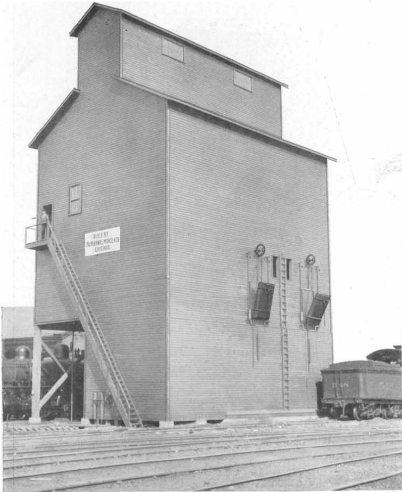
Coaling Station at Raleigh, N. C., on Seaboard Air Line. Storage capacity, 850 tons.
