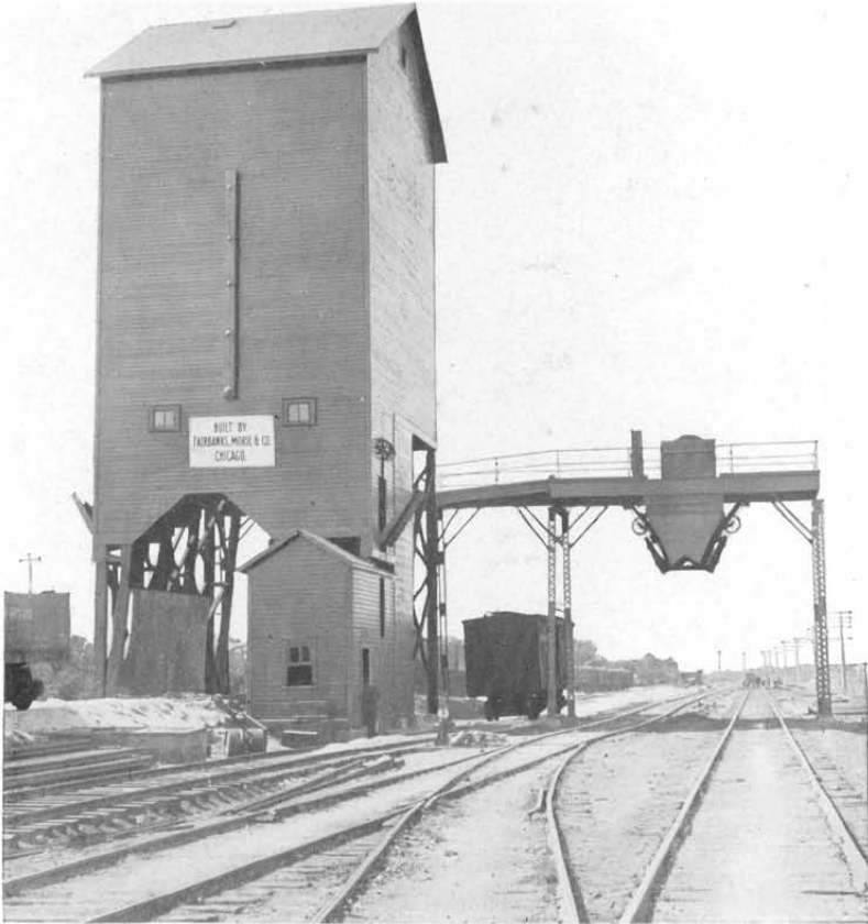
Coaling Station at Florence, Kan., on A. T. & S. F. Ry. Storage capacity, 300 tons. Coal is weighed in Fairbanks Standard Hopper Scales.
