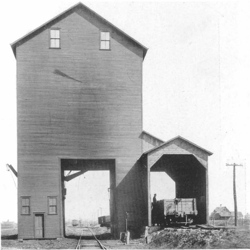
Coaling Station at Port Huron, Mich., on Pere Marquette Ry. Storage capacity, 160 tons. We have erected twelve similar coaling stations for this road.
