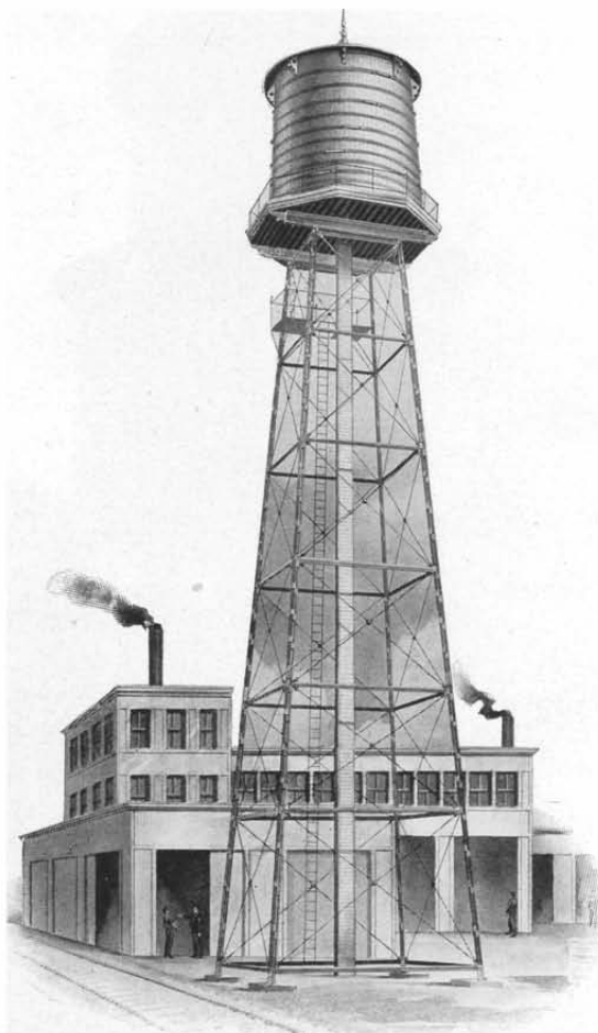
20 x 18-foot Tank on 90-foot Steel Tower
