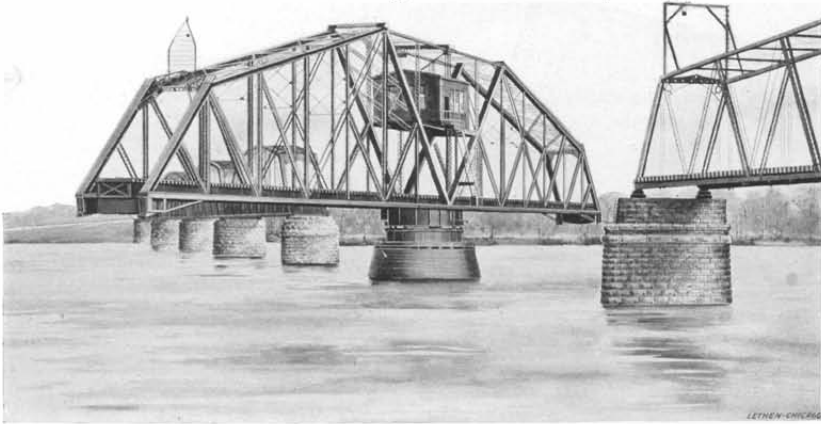
Drawbridge on L. & N. R. R., Danville, Tenn., operated by 28 H. P. Fairbanks-Morse Gasoline Engine. Length of span, 400 feet. Weight of draw, 1,250,000 pounds.
