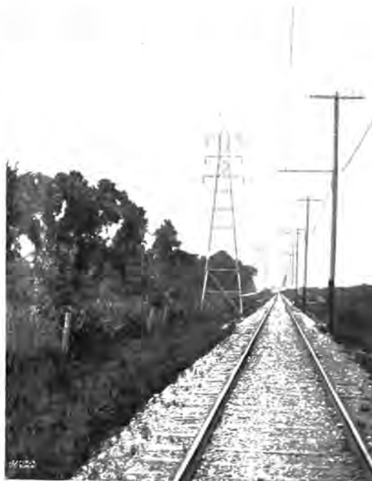
Fig. 18 VIEW OF TRANSMISSION, TROLLEY AND FEEDER LINE, SHOWING BRACKET CONSTRUCTION
