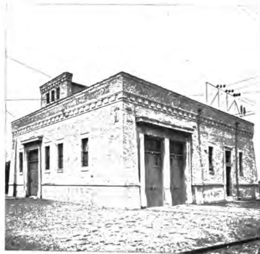
Fig. 7 EXTERIOR OF BURLINGTON AND WAUKESHA SUBSTATION
