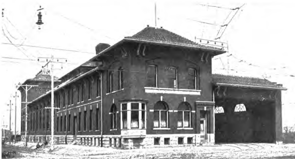
Fig. 9 EXTERIOR OF WEST ALLIS SUBSTATION
