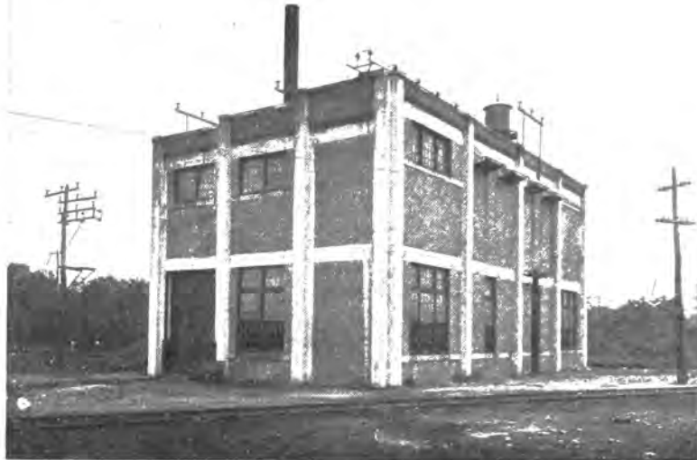
Fig. 11 NAVAL ACADEMY SUBSTATION
