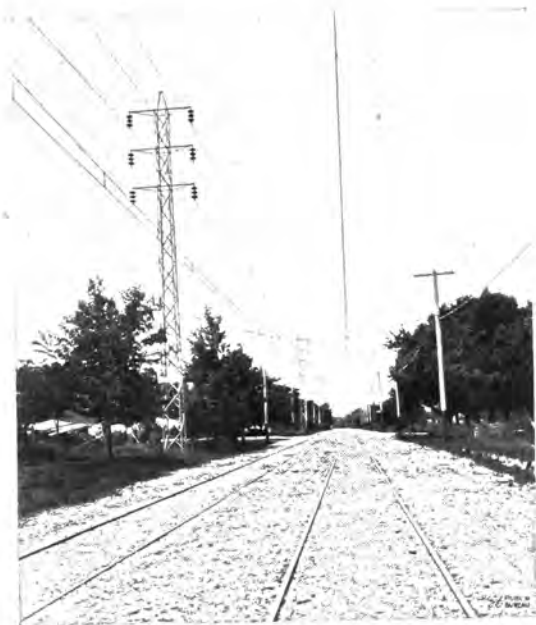
Fig. 17 HIGH TENSION TRANSMISSION TOWER USED IN CITIES AND TOWNS
