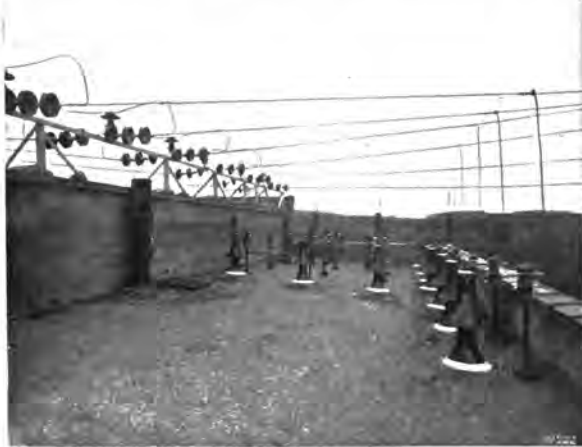
Fig. 19 TAPPING TRANSMISSION LINE ON SUBSTATION ROOF
