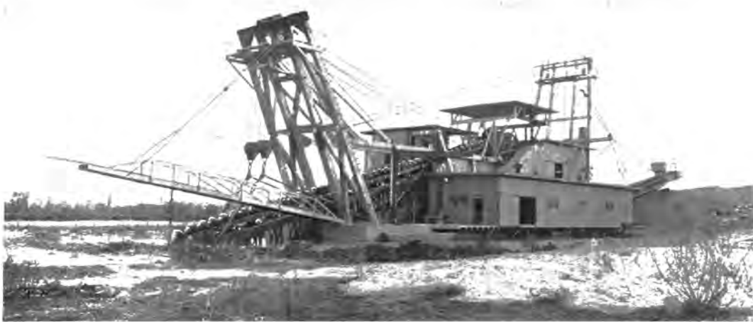
GOLD DREDGE YUBA NO. 12, MARYSVILLE, CAL., ELECTRICAL EQUIPMENT IS THE SAME AS THAT OF YUBA NO. 11 SHOWN ON PAGE 3
