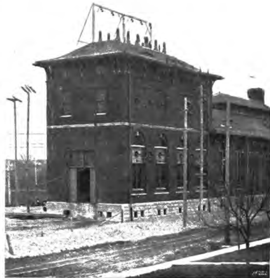
Fig. 8 EXTERIOR OF WEST ALLIS SUBSTATION
