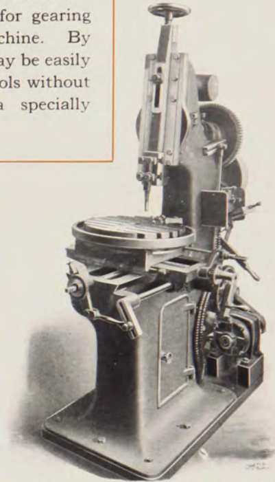
NILES-BEMENT-POND CO. 6-IN. SLOTTER DRIVEN BY KT-4, 2 H.P., 1800 R.P.M. INDUCTION MOTOR
