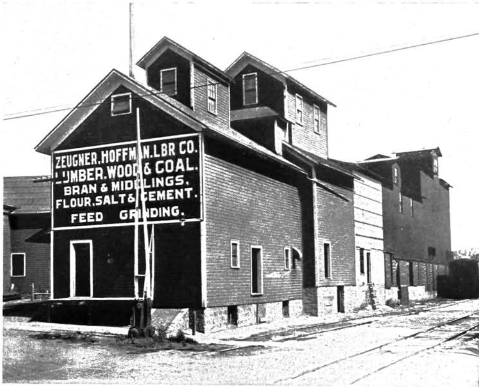
ELEVATOR AND MILL BUILDINGS
