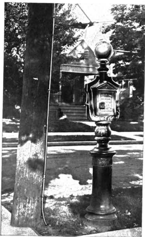
FIRE ALARM BOX IN ROCHESTER, N. Y., LIGHTED FROM SL TRANSFORMER
