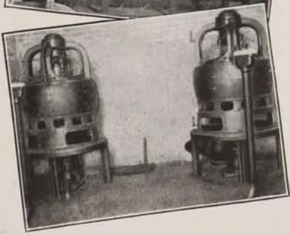
50 h. p. vertical type pump motors.
