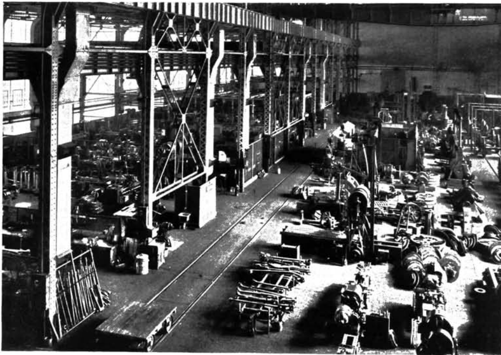
GENERAL VIEW OF MACHINE SHOP, LOOKING EAST
