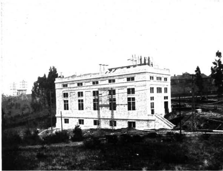
OAKLAND SUBSTATION, GREAT WESTERN POWER COMPANY
