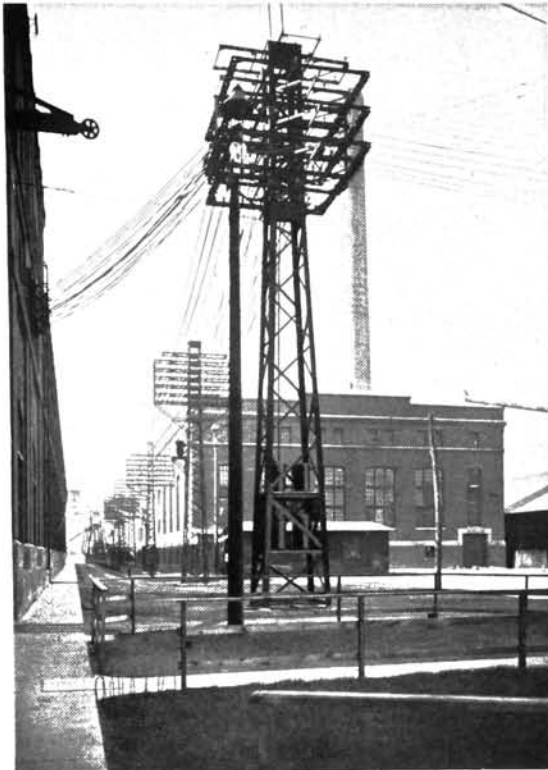
VIEW LOOKING SOUTH SHOWING STEEL TOWER TRANSMISSION LINE, WITH POWER HOUSE IN BACK GROUND, AND WEST END OF MACHINE SHOP AT THE LEFT
