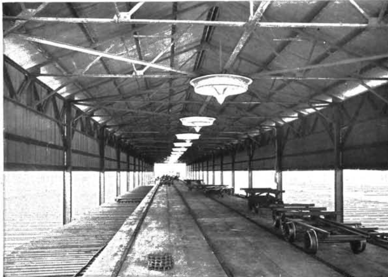
SHED USED FOR THE GRADING OF KILN DRIED LUMBER. LIGHTED BY GENERAL ELECTRIC ENCLOSED ARC LAMPS FITTED WITH LIGHT BALANCING CEILING DIFFUSERS—THE GREAT SOUTHERN LUMBER CO., BOGALUSA, LA.
