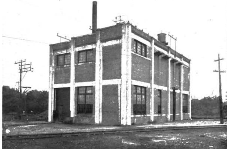
Fig. 11 NAVAL ACADEMY SUBSTATION
