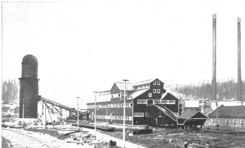
WOOD BURNER, MILL, POWER STATION AND LOG POND, ELK RIVER MILL
