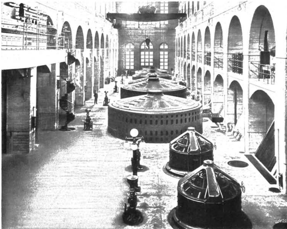
10,000 AND 7500 KW. GENERATORS AND 400 KW. EXCITERS IN THE PENNSYLVANIA WATER AND POWER CO'S STATION, MC CALL FERRY, PA.
