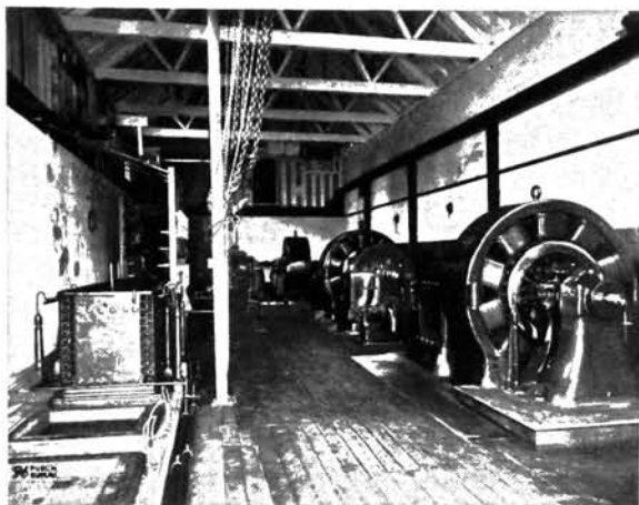
TY GENERATORS IN THE FIRST THREE-PHASE TRANSMISSION PLANT
