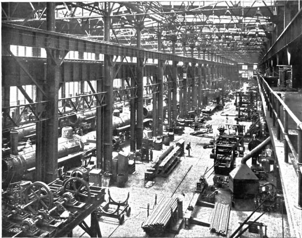
PORTION OF MACHINE SHOP ON THE RIGHT; ERECTING SHOP ON THE LEFT
