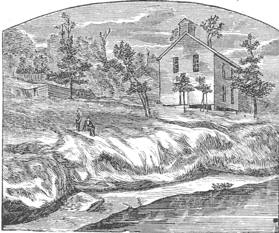
BAPTIST CHURCH AND MASONIC HALL.
